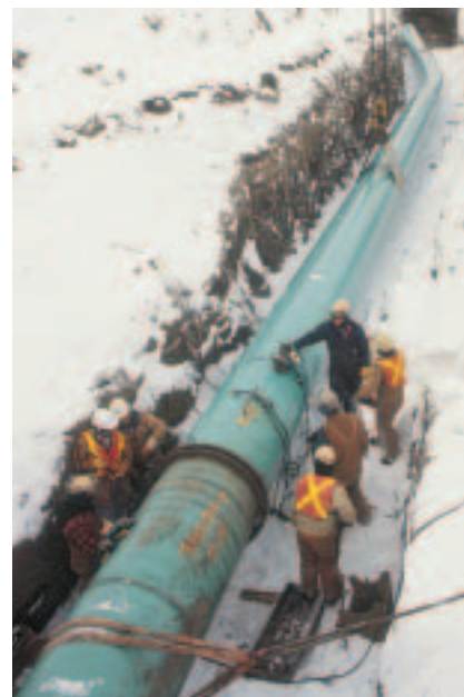
Figure 2.17b) Workers installing a gas pipeline
