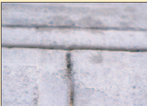
Figure 2.19c) Did you ever notice that sidewalks are made of slabs with gaps between them? What is the advantage of leaving these gaps? What might happen if the slabs were placed right up against each other?
